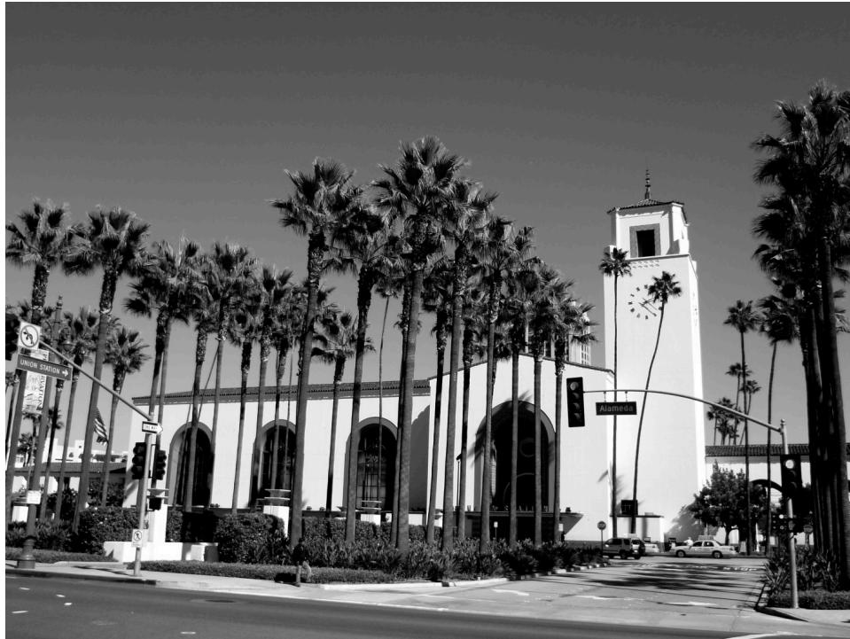
Figure 1: Exterior of Union Station West, showing the clock tower and the main entryway
